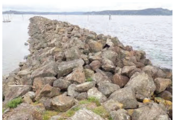
Photograph 6 Rubble mound breakwater
