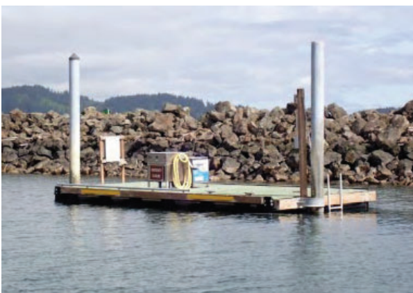
Photograph 5 Sewer pumpout float
