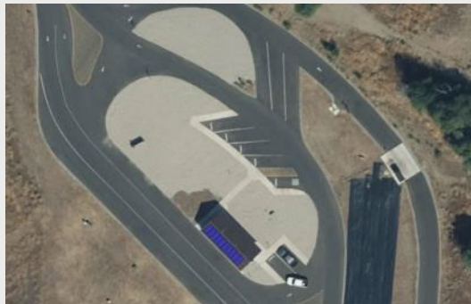
Pearrygin L. Contact Station Rooftop Array: 5.0 kW Cost per Watt = $10.80
