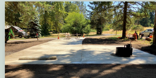
ADA Campsite Renovation
