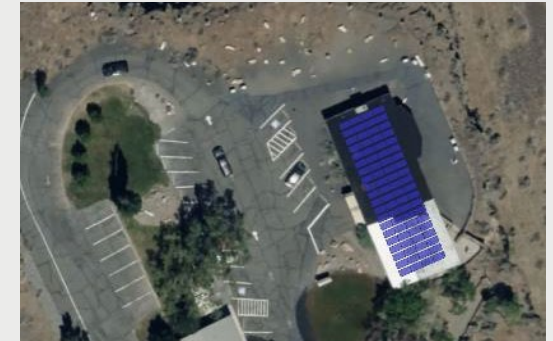
Ginkgo Petrified Forest IC Rooftop Array: 44.0 kW Cost per Watt = $11.20
