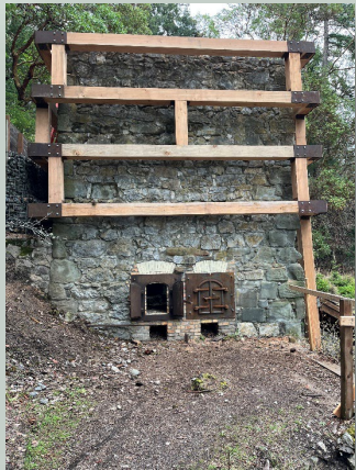
Restoration of Lime Kiln on San Juan Island
