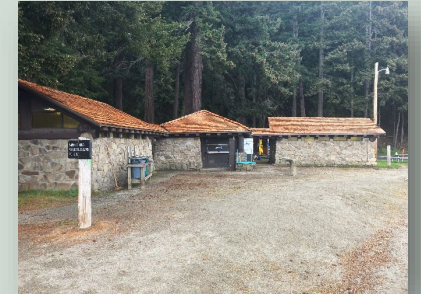
Historic Buildings Re-Roofing
