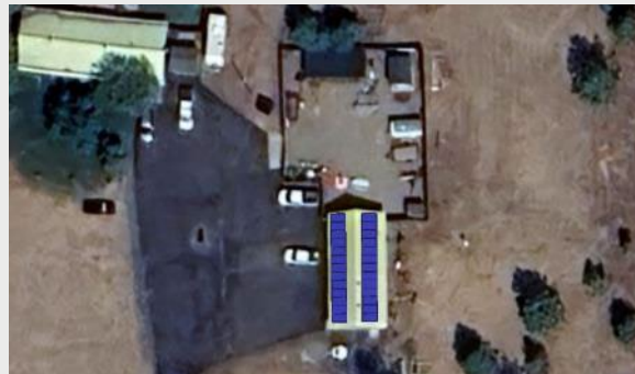
Riverside – ORV Shop Rooftop Array: 14.0 kW Cost Per Watt = $11.10
