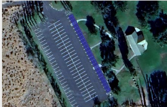
Ginkgo-Wanapum parking Carport Array: 76.0 kW Cost Per Watt = $18.30
