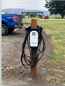
EV Charging Station Installation
