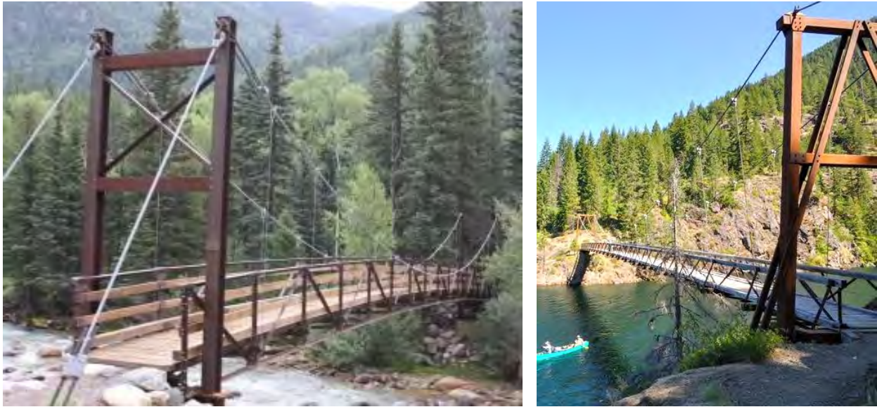
Figure 22: Example of suspension-style trail bridges
