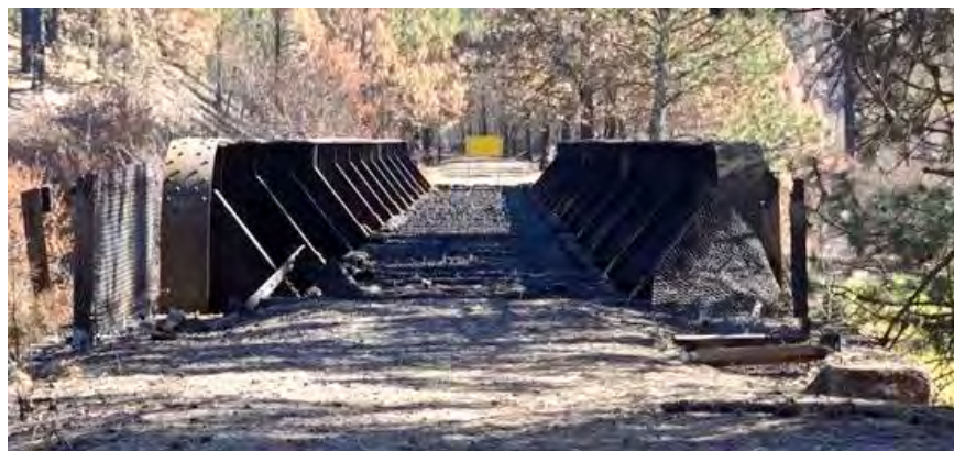
Figure 16: Pine Creek Bridge, Palouse to Cascades Trail
