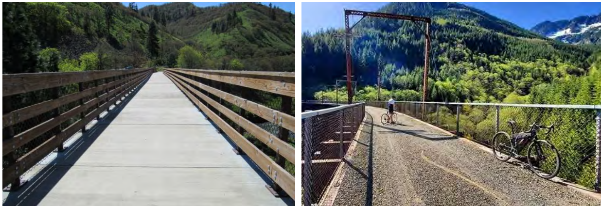
Figure 13: Fisher Hill Rd Bridge along Klickitat State Park Trail with concrete deck (left) and Mine Creek Trestle along Palouse to Cascades Trail with aggregate overlay (right)
