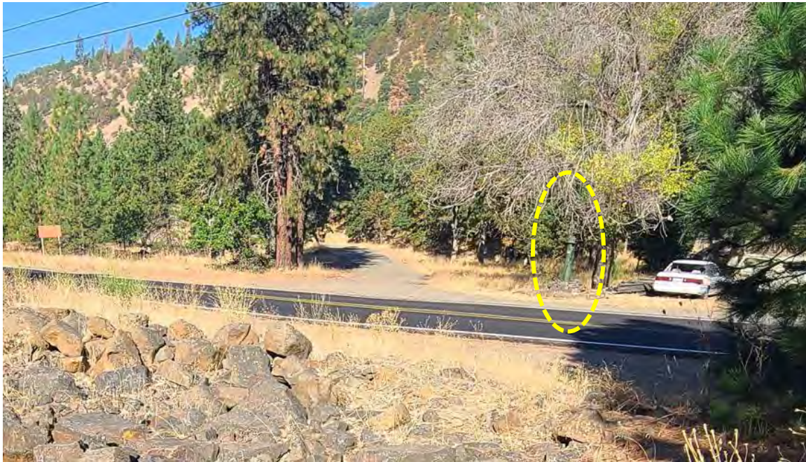
Figure 10: Standpipe north of Suburbia Crossing at SR 142 (looking north).
