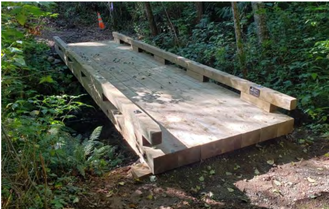
Figure 25: Example of timber prefabricated bridge
