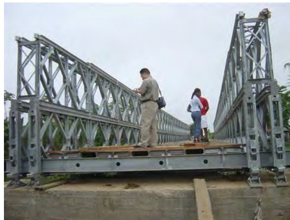
Figure 19: Example of through-truss bridge
