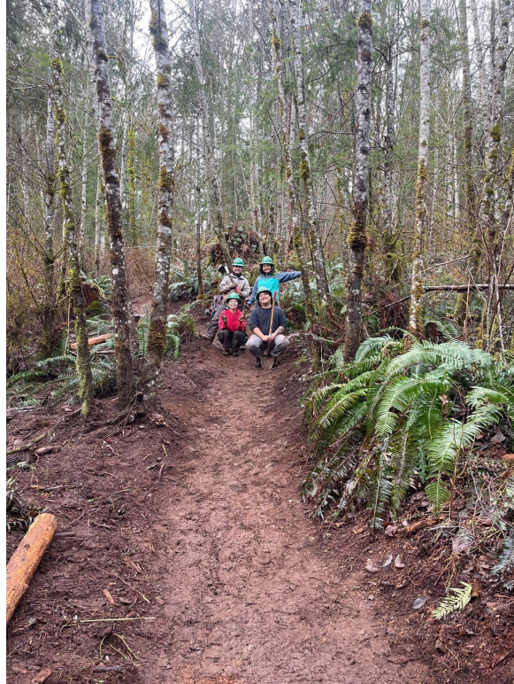
New Trail Construction
