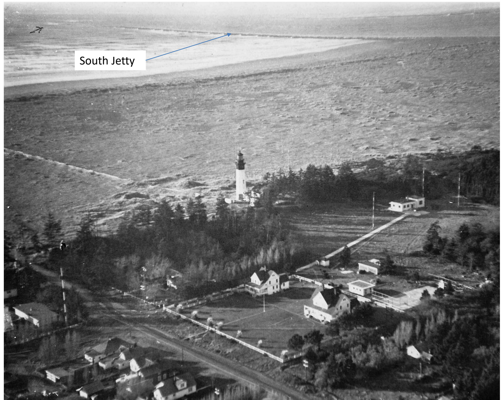
Construction of the south jetty began in 1898, which resulted in an approximate 3000-foot horizontal westward expansion of the existing shoreline.
