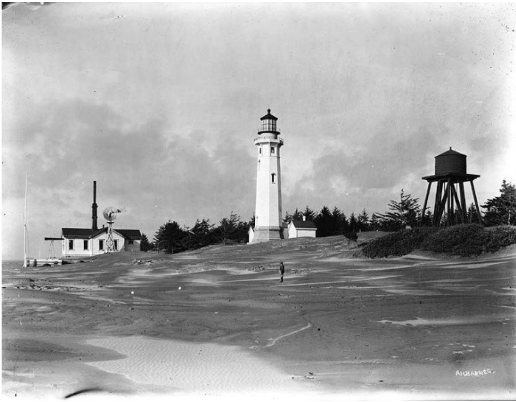
The Lighthouse (Life-Saving Station) was constructed in 1897 with light and fog signals along the beach.
