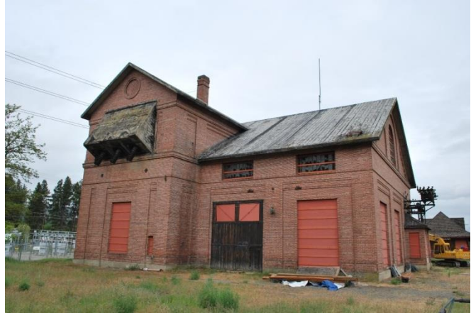
Substation, South Cle Elum Railyard
