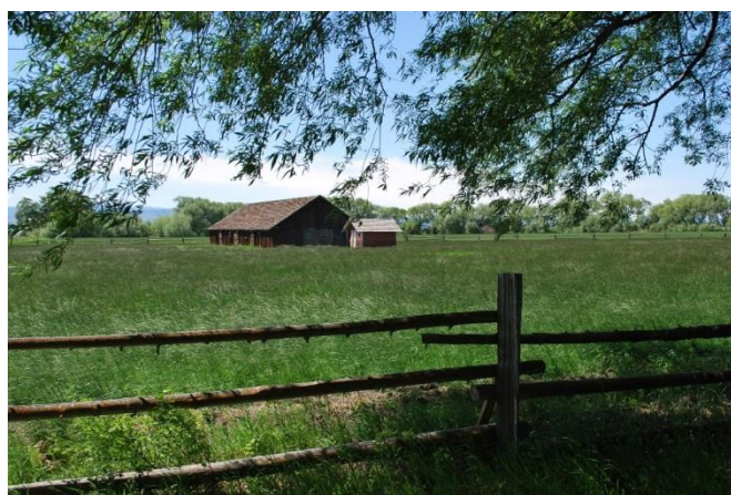
Dairy Barn, Olmstead Place
