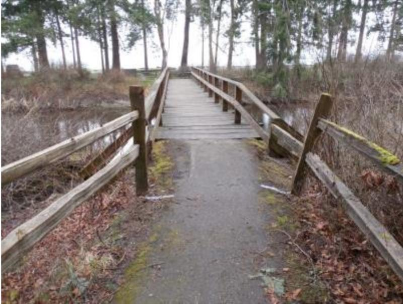
**Footbridge One (Facing east – the white line marks the center of the new concrete abutment)**
