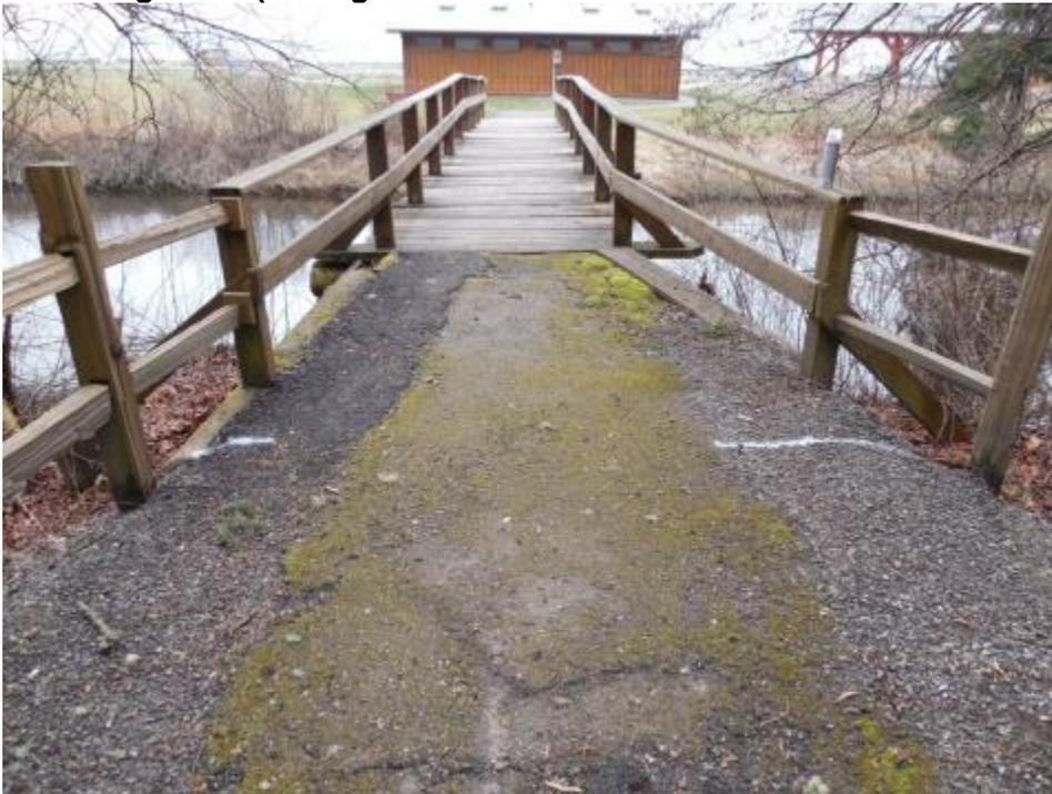
**Footbridge Two (Facing east – the white line marks the center of the new concrete abutment)**
