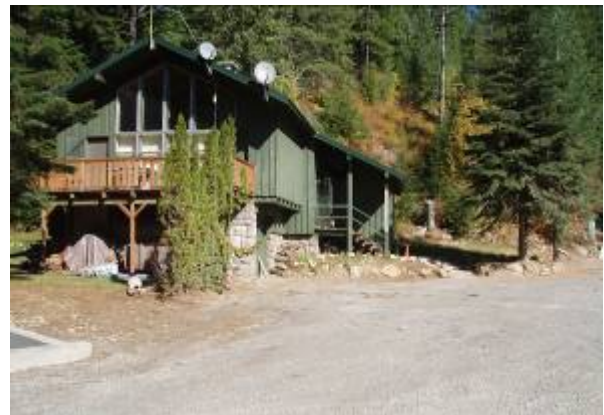
The existing park residence has the potential to serve as a year round gateway orientation center.
