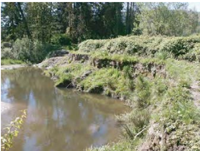
Revegetation would stabilize the existing streambank
