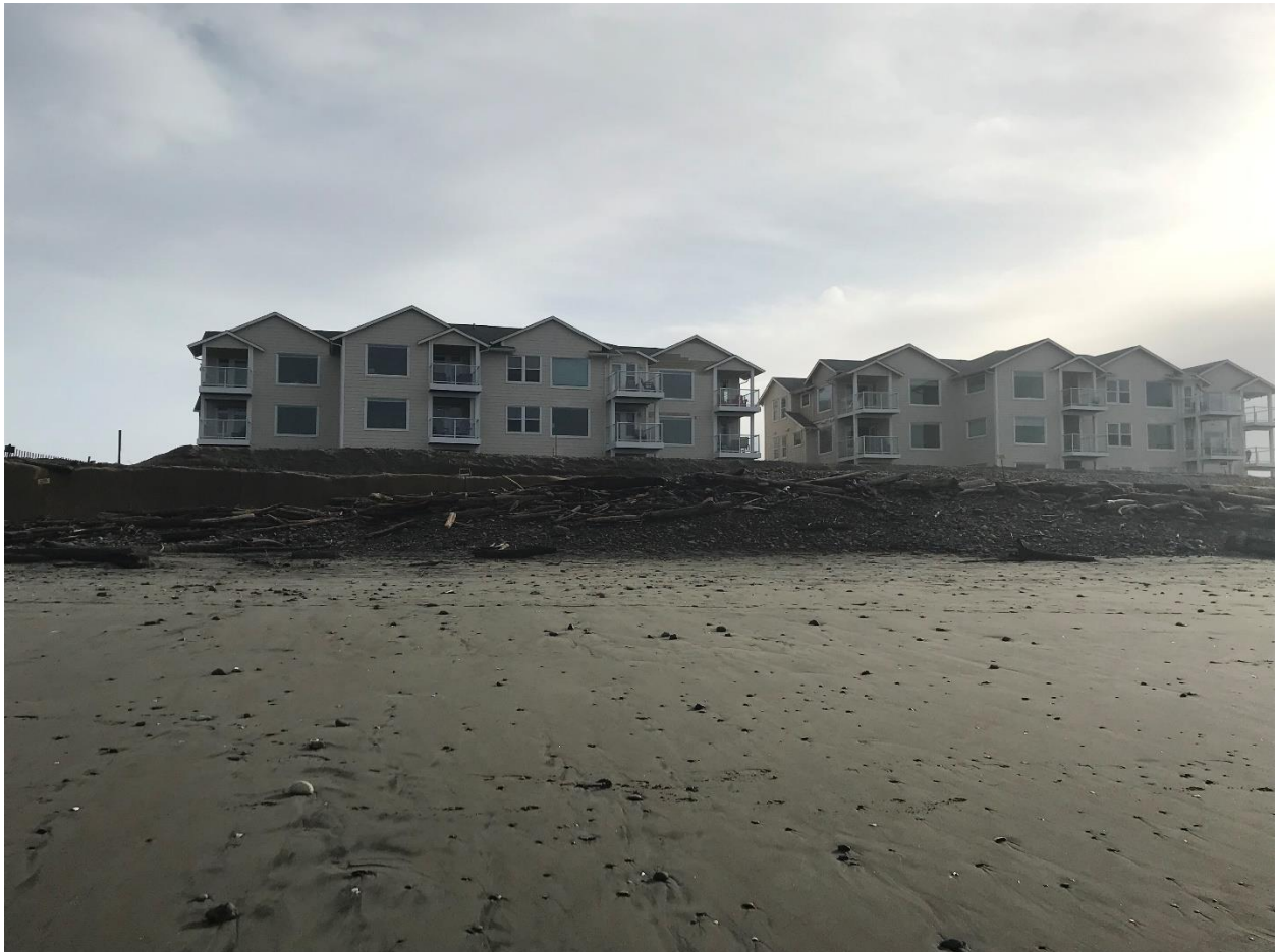
Figure 5. Long-term retreat of the beach and dunes has threatened the Westport by the Sea Condominiums, immediately south of the Westport Light State Park boundary. A dynamic revetment was built in December 2021.
